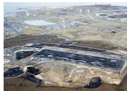
Above Aerial view of the Laggan-Tormore gas plant project on the Shetland Islands, UK.
